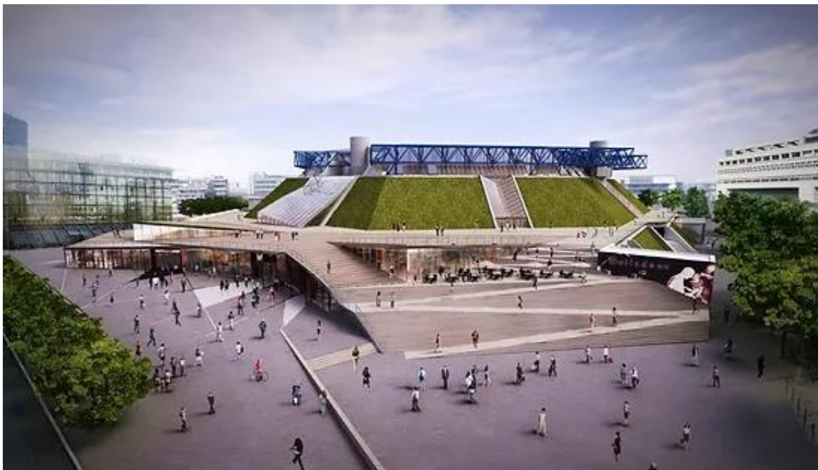
Renovation of the Hotel accord Aréna Paris Bercy https://www.dvvd.fr/projet/accorhotels-arena
