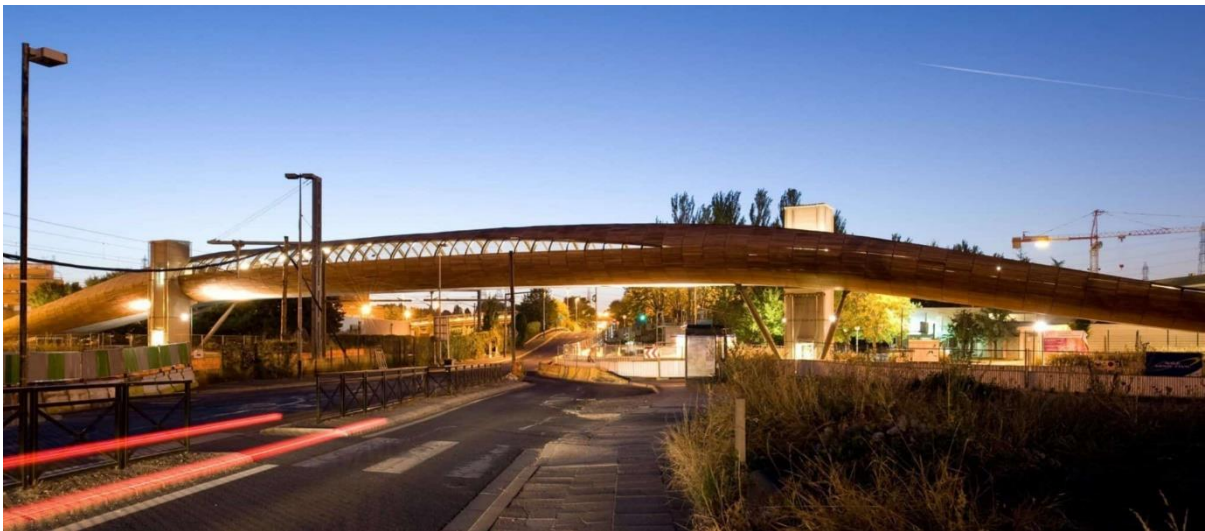
Footbridge in Villetaneuse
