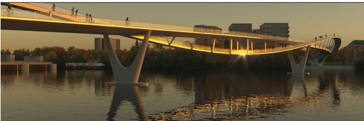
Footbridge over the Neckar in Hedelberg
